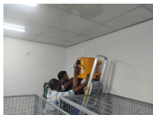
Infrastructural renovation of single-shop LBM
