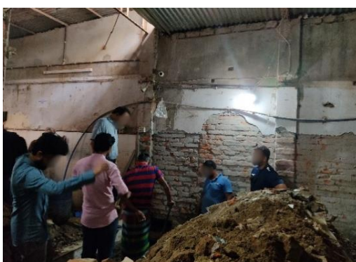
Infrastructural renovation of single-shop LBM
